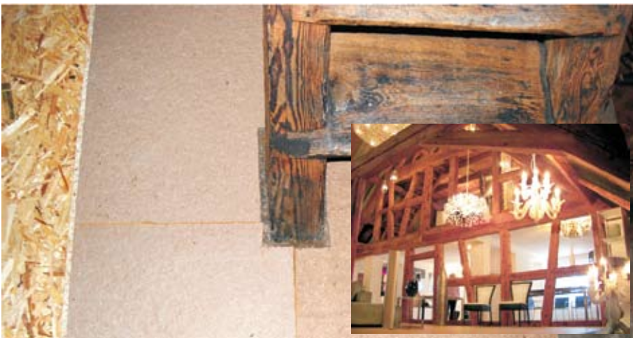
Old house sanation with hofafloor.
